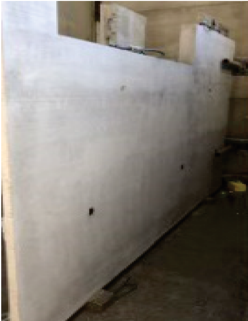
Type 'C' Finish at 5 Meter's Internal Wall
