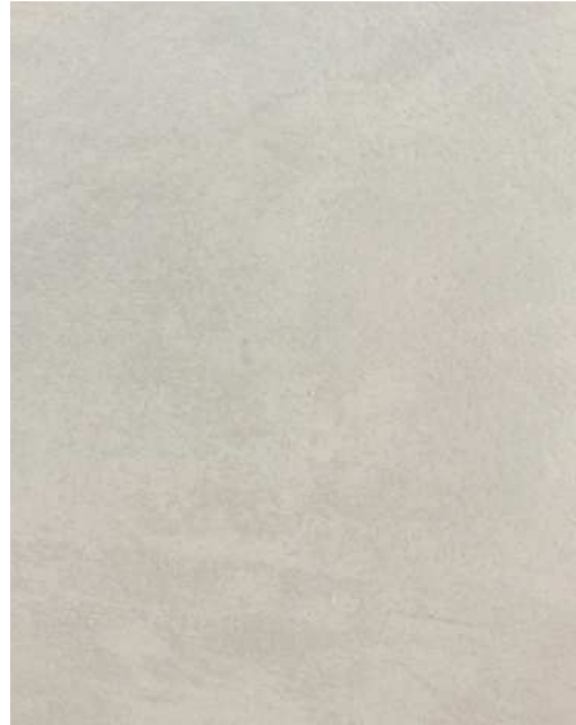
Type 'C' Finish at 1 Meter's Internal Wall
