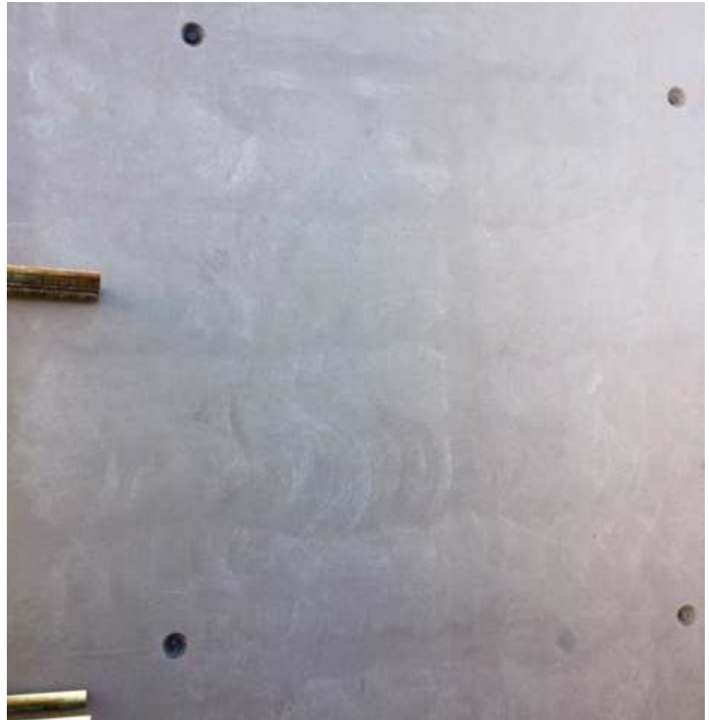
Type 'B' Finish at 1 Meter's Internal Wall
