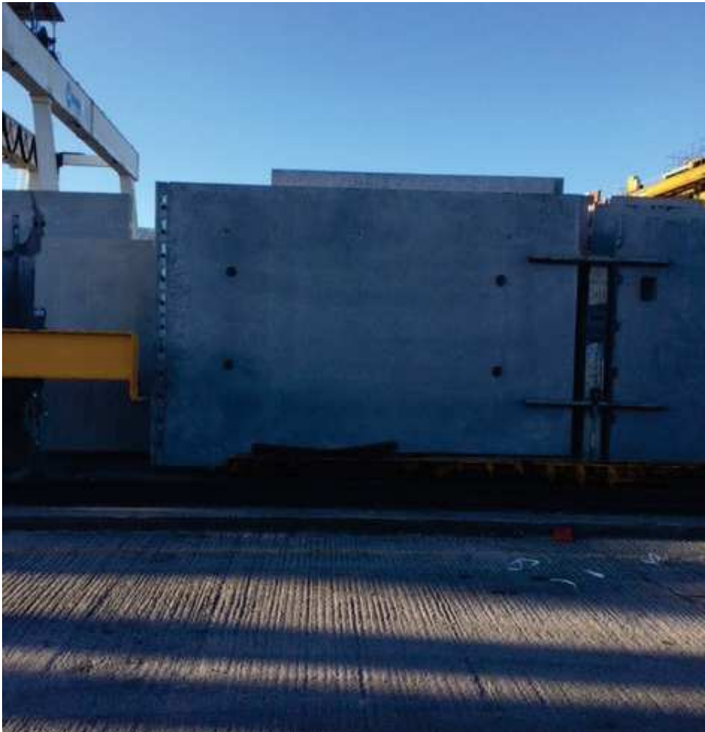
Type 'B' Finish at 5 Meter's Internal Wall
